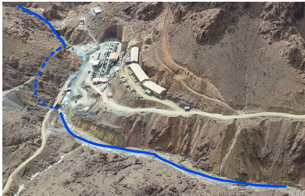
Other view of the cyanide processing plant, with the Zgounder river nearby. The dark blue line is the current riverbed of the Zgounder river, including the underground deviation. The light dotted line is the old riverbed before deviation.
