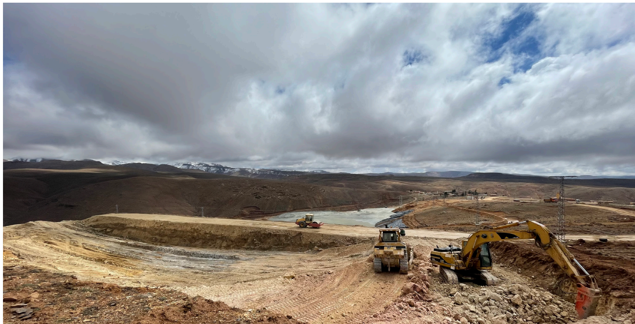
Earthworks in preparation for the construction of a 30,000m 3 water basin
